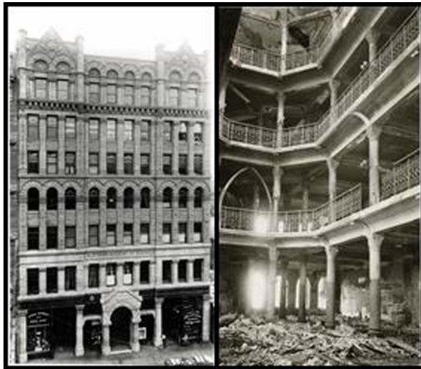
FIGURE 5. Views of the California Academy of Sciences building, including, (left), before fire and (right), after fire in 1906. Courtesy of the California Academy of Sciences Library.
